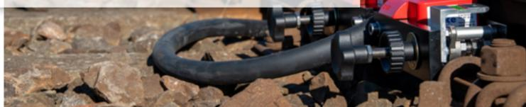
The axle counter detects arriving trains and forwards the signal to the base station.
