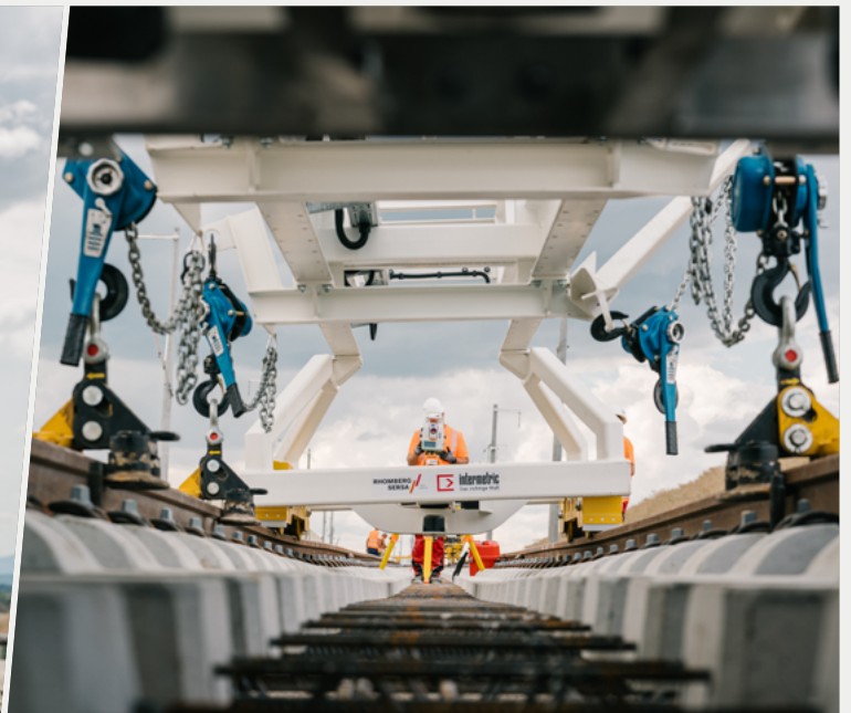
Support for the construction of slab tracks
