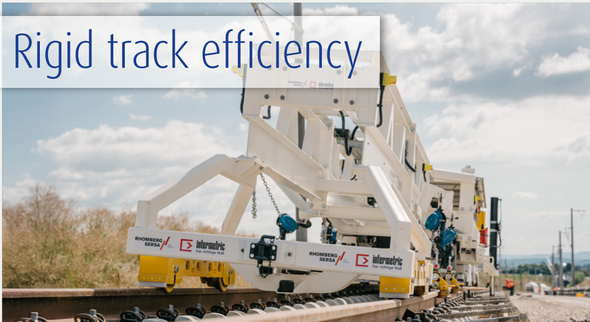
RhoMAT combines several work steps and simultaneously increases the accuracy of the end product
